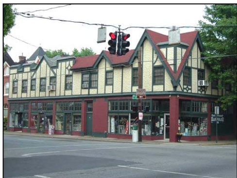
A view of the northeast corner of 4 th & Oak Streets
